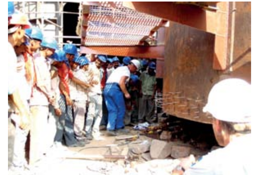
Participation in the ceremonial blessing of the digester top.
